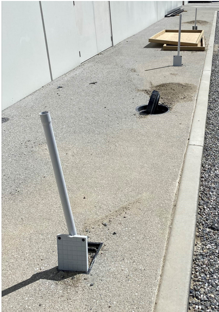
Installation of Pedestal supply pits for future use
